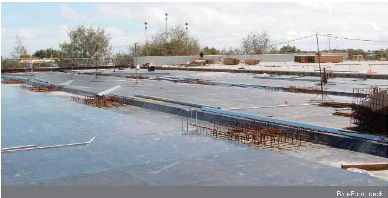
BlueForm in use as part of a form deck
