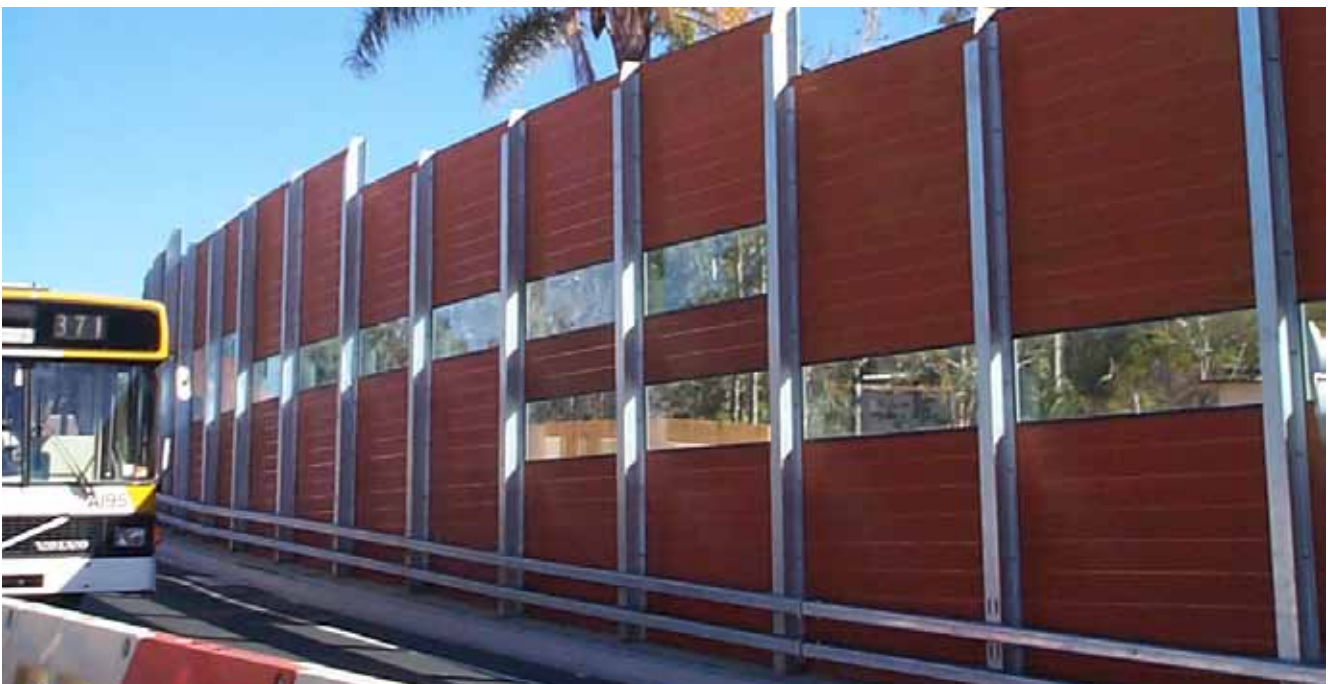
EzyShield Commercial used in a freeway application
