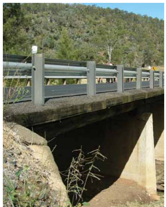
Completed BridgeDeck project
